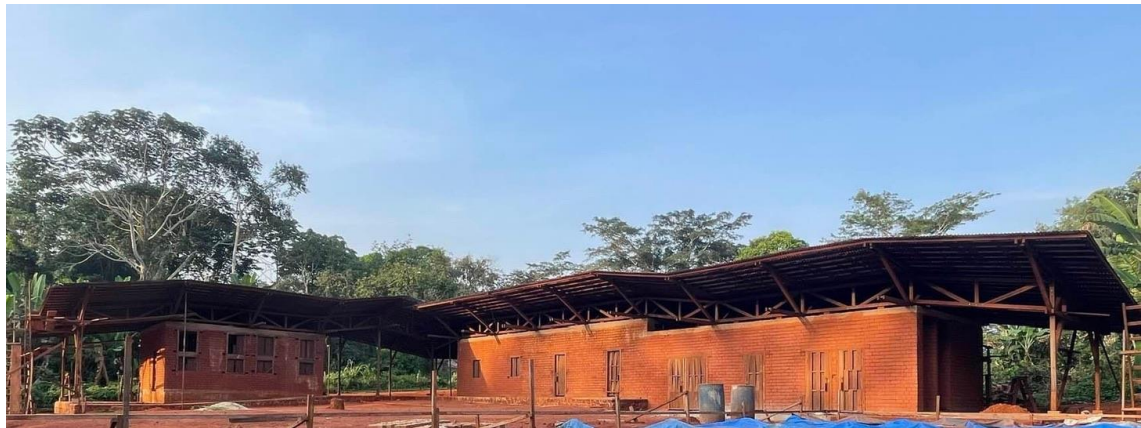
Figure 2: Zoulabot Field Station under construction
