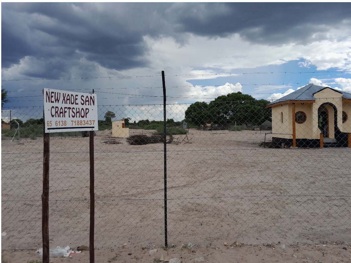
Photo 1: Exterior view of the New Xade San Craftshop
