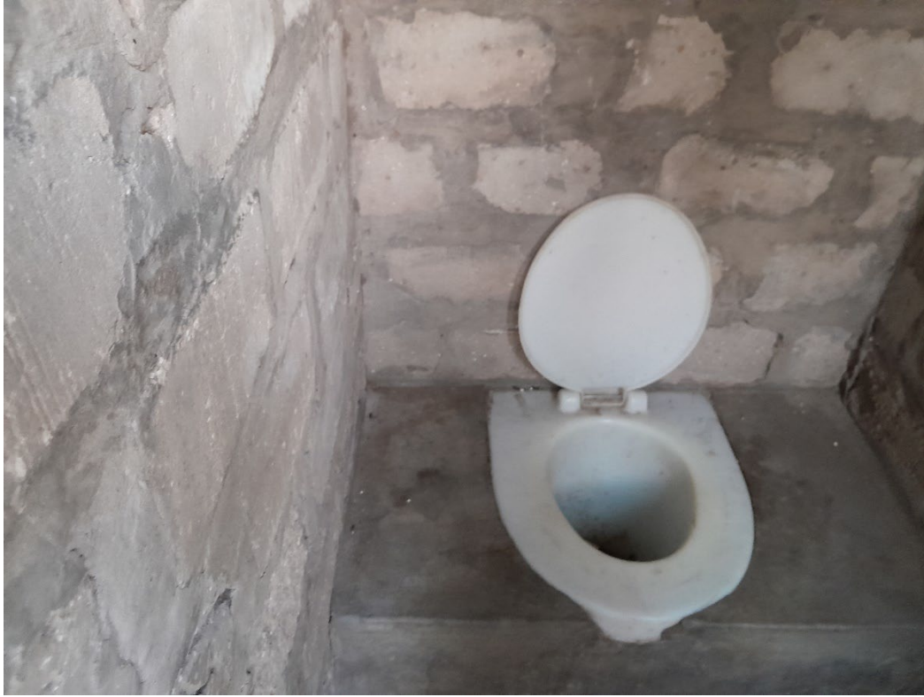
Photo 3: Toilet in New Xade Village (2).
